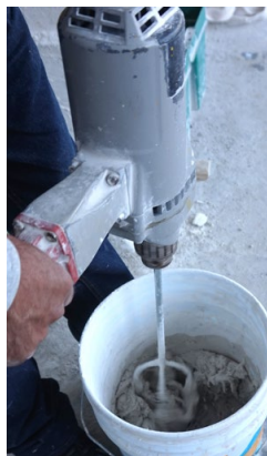
Figure 8 Mixing Litecrete Mortar
